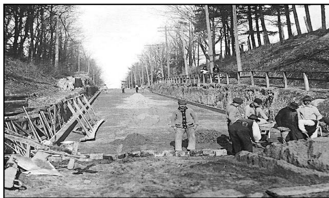
Smoothing out the Dufferin Street hill north of Davenport, 1912.
